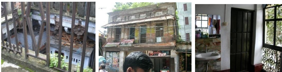
Figure 2: Types of transformation in Old Dhaka (L-R) - courtyard, the center for domestic activities and spatial composition, a space for further addition and subdivision; verandas converted to storage or additional bed room; conversion to shop-houses.
