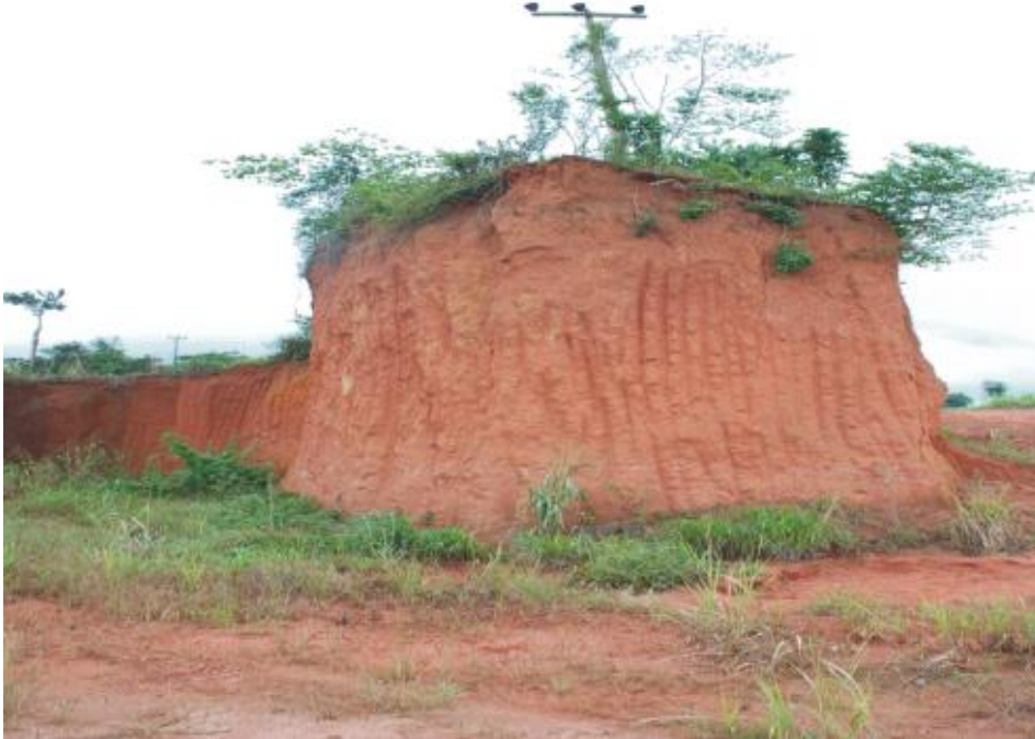
Plate 2: Excavation that endangered Electric Pole
